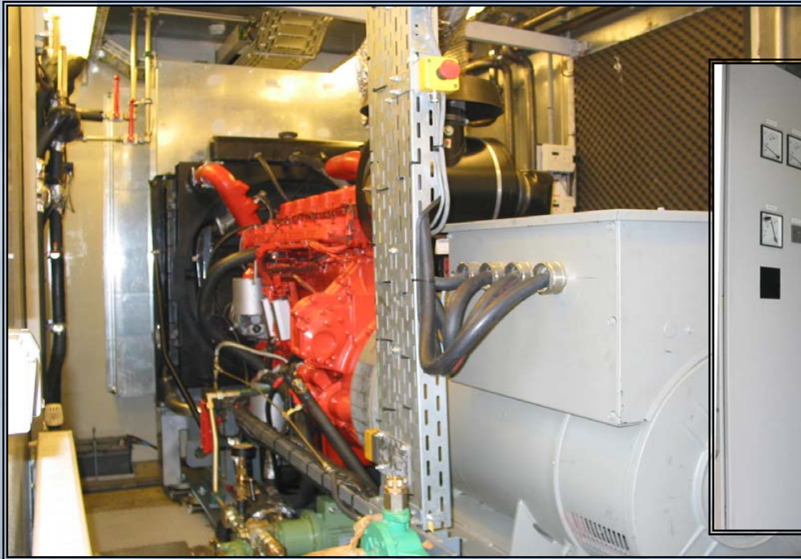
Containerized Cogeneration Unit & Switchboards for vegetable oil
