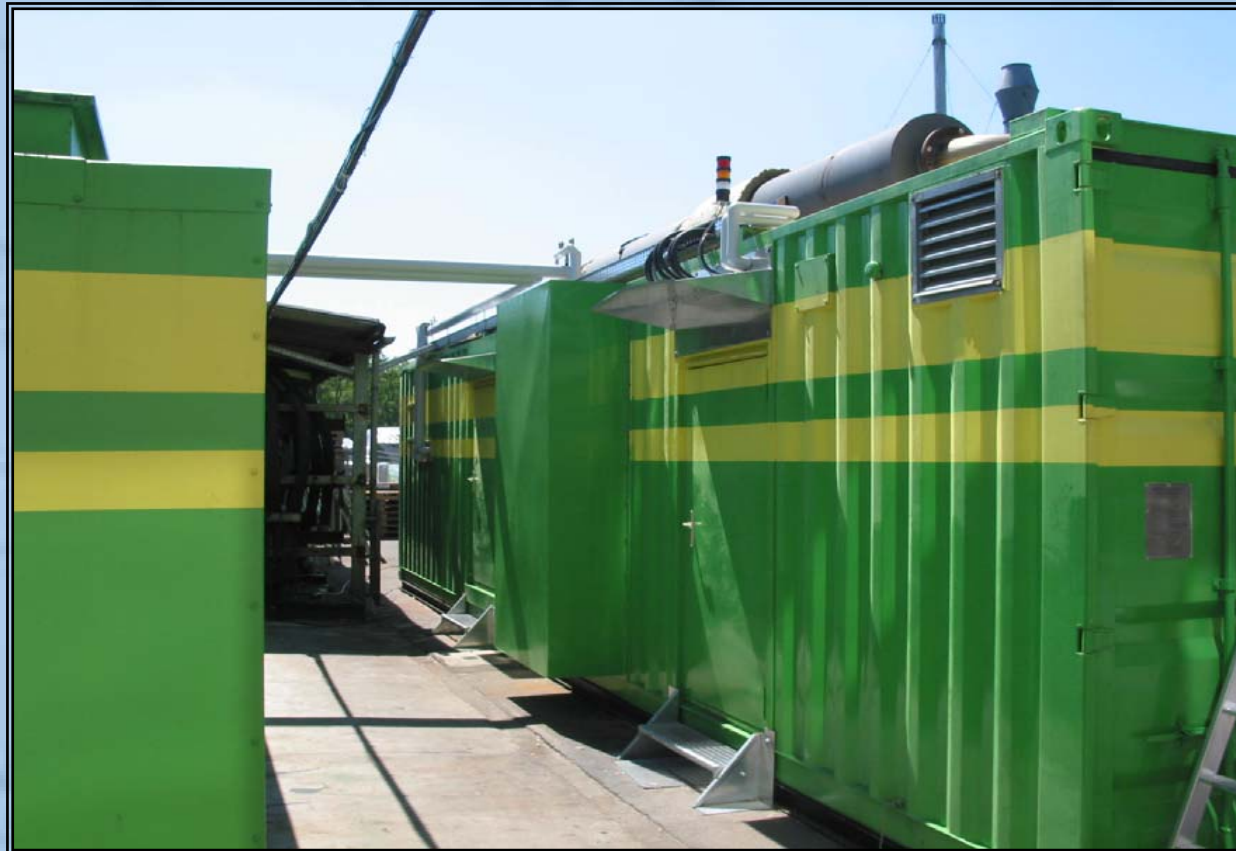
Container for Cogeneration Unit (vegetable oil) 210 kWel
