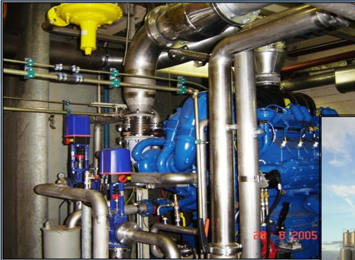
Compressor Drive for Food Industry in Germany (350 kW, Deutz)
