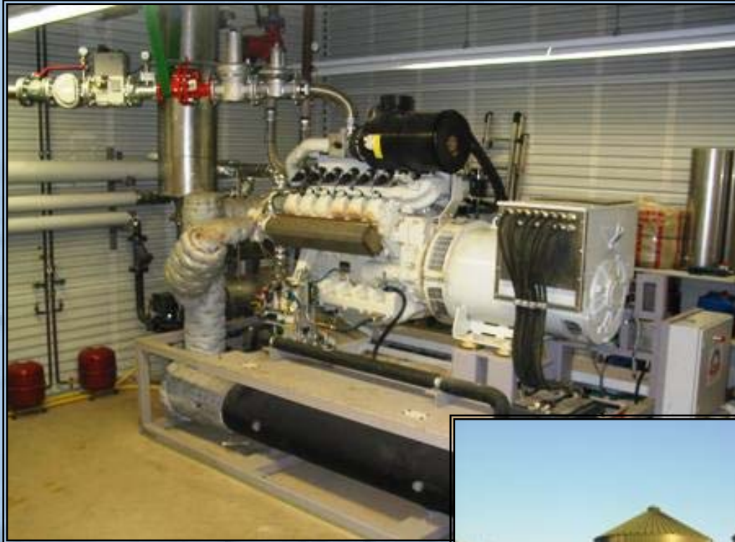
CHP (2 x 347 kW, MAN) for Biogas in Bersenbrück (Germany)
