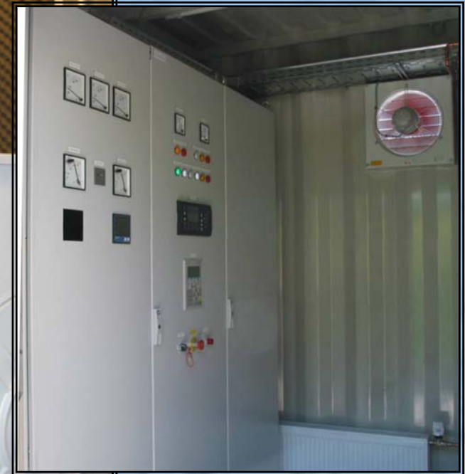
Containerized Cogeneration Unit & Switchboards for vegetable oil
