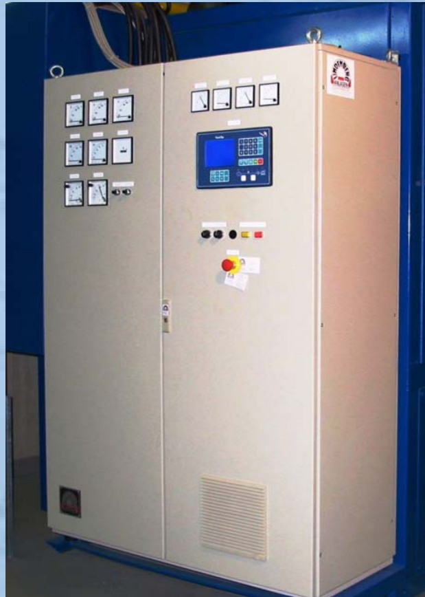
Switchboard for Cogeneration Unit
